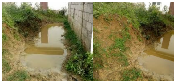
Figure 3: water accumulation due to poor drainage system
