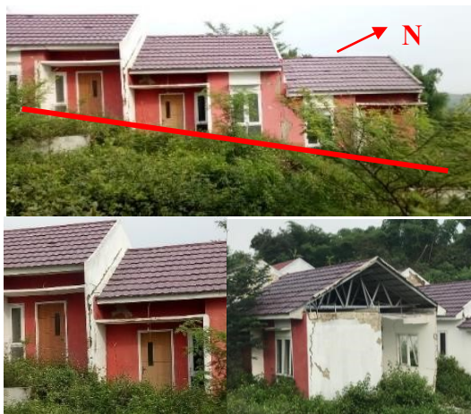
Figure 2: Housing is built on sloping land with damaged house walls
